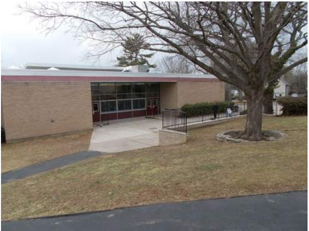
Existing Student Entry
